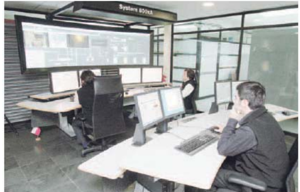
Remote diagnostic room at ABB offices in Santiago-Chile
